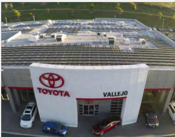
Toyota of Vallejo installed a 251 kW rooftop solar system that is offsetting an average of 61 percent of the dealership's electricity needs.
