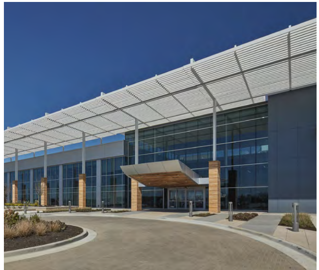
The new Toyota Production Engineering and Manufacturing Center in Georgetown, Kentucky
