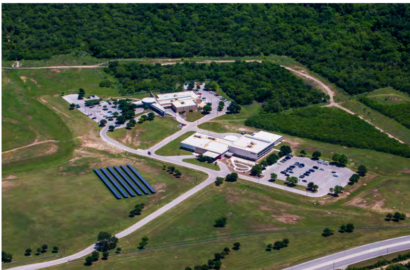
Toyota’s assembly plant in San Antonio, Texas, installed a 200-kilowatt ground-mount solar array to support the Visitor and Education Center and the Family Health Center.
