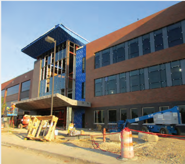
During the construction of Toyota's new R&D campus in York, Michigan, 461 tons of material were diverted from landfill. That's 92 percent of construction waste put to productive use.
