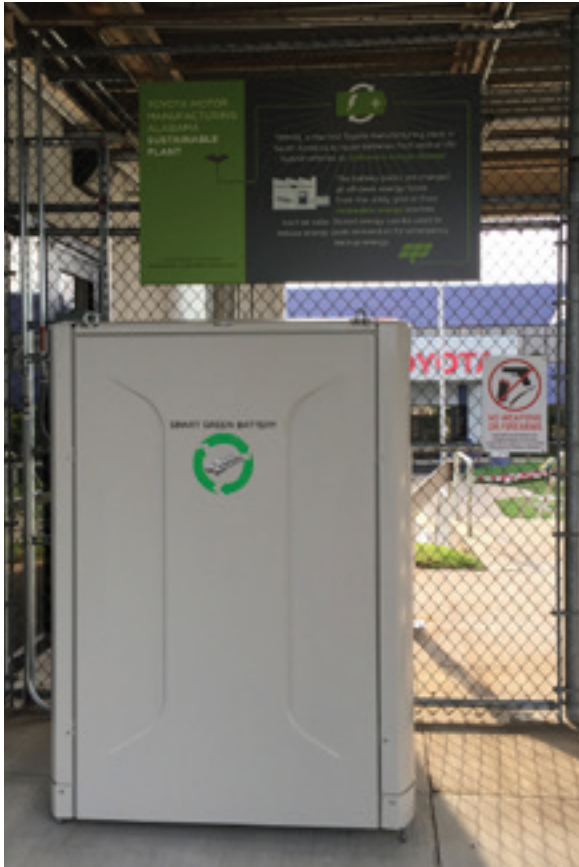
Toyota Motor Manufacturing, Alabama (TMMAL) is the first Toyota manufacturing plant in North America to reuse batteries from end-of-life hybrid vehicles as stationary energy storage.
