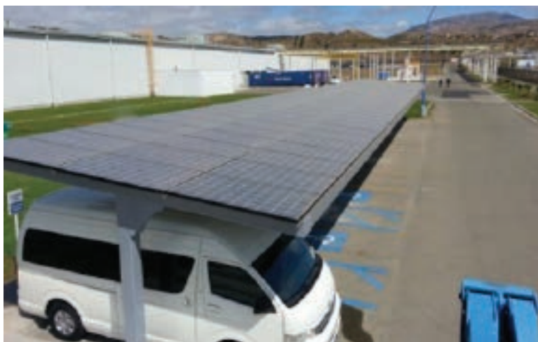
The new photovoltaic (PV) carport at Toyota's assembly plant in Tecate, Mexico, generates up to 121 kilowatt hours of renewable electricity each day – equivalent to the daily energy requirements of about 15 typical Tijuana-area homes.
