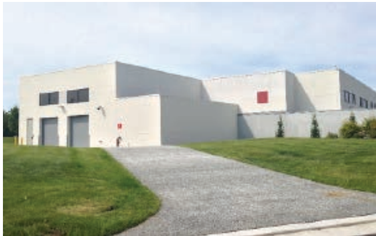
With the expansion of our Technical Training Center in Glen Burnie, Maryland, we are getting a jump on the 2015 launch of our fuel cell vehicle. This center integrates special features to allow for an easy transition to hydrogen vehicle service.
