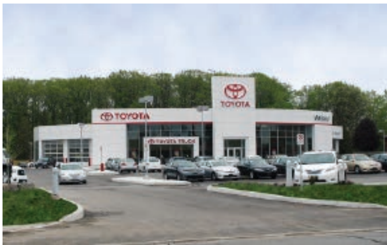
Welland Toyota is our third LEED-certified dealership in Canada. It earned Gold certification by incorporating a host of green elements to reduce energy and water use, recycle, and reduce waste going to landfills.
