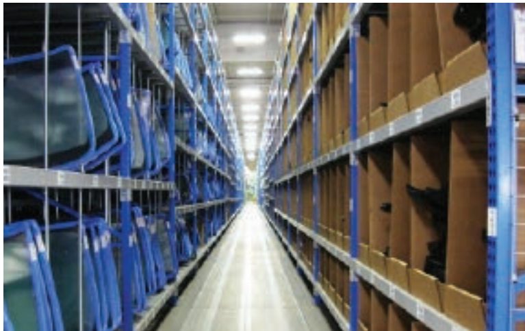
An example of the difference in lighting quality as a result of a lighting upgrade is shown above. After upgrading, the lighting at the Los Angeles Parts Distribution Center is brighter without requiring more energy use, and the individual fixtures are now controlled by motion sensors.
