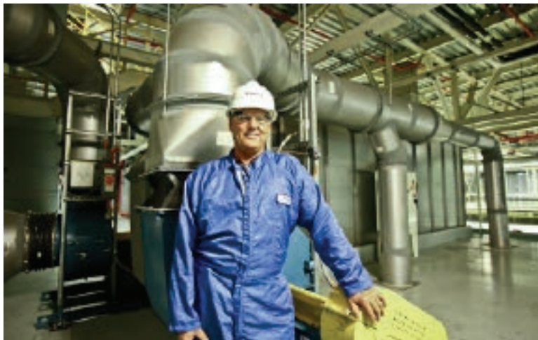
Paul Houchins is a paint specialist at Toyota Motor Manufacturing, Indiana. He has been working on making the system that conditions air for the paint booth more energy-efficient. His breakthrough came when he realized the conditioned air in the plant’s general assembly area could be captured and used in the paint booths before being expelled by exhaust fans. This reduces the need to draw in fresh outside air by 40 percent. The result is a reduction in natural gas consumption, which decreases the Indiana plant’s CO 2 footprint by over 7,700 pounds a year. The savings is equivalent to the amount of carbon sequestered annually by 2.9 acres of U.S. forests.
