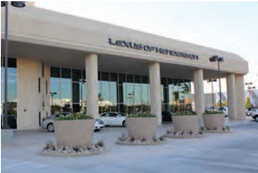
Lexus of Henderson in Nevada is the third Lexus dealership to receive LEED Gold certification. Thanks to a number of green building strategies, this dealership has reduced energy use by 38 percent and water use by 42 percent.
