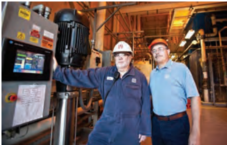
Rob Coveney and John Goodfellow are two of the engineers at our manufacturing plant in Cambridge, Ontario, who helped to develop a reverse osmosis concentrate recovery system that is saving the plant over 50,000 cubic meters (13.2 million gallons) of water annually.
