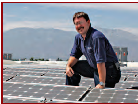
Our parts center in Ontario, California, installed a photovoltaic array that is expected to produce more than 3.7 million kilowatt-hours per year. This provides almost 58% of the electricity needed at the facility.
