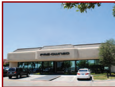
2009 The pre-owned building of Sewell Lexus of Fort Worth, Texas, is the first Lexus dealership to achieve LEED certification.
