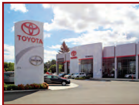
2010 The Kendall Toyota dealership in Eugene, Oregon, achieves LEED Platinum, the highest level of certification possible and the first LEED Platinum dealership in the world.
