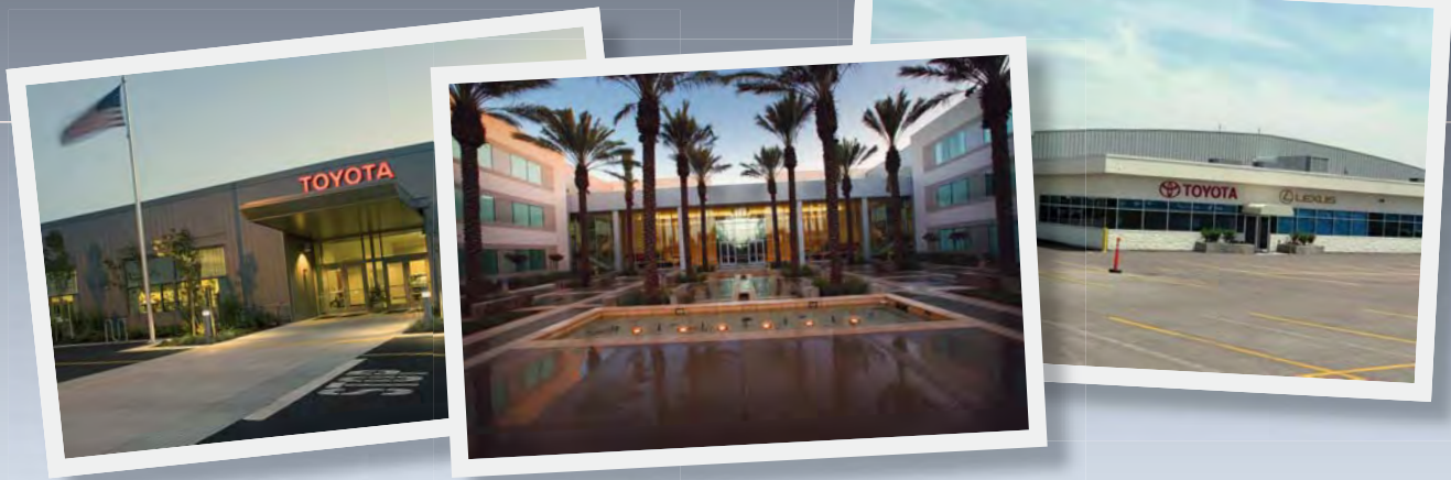
Three of Toyota's sales and logistics sites used a number of sustainable practices during construction or renovation: the Port of Portland Vehicle Distribution Center, the South Campus of Toyota Motor Sales, U.S.A. headquarters in Torrance, California, and the Toronto Vehicle Processing Center.
