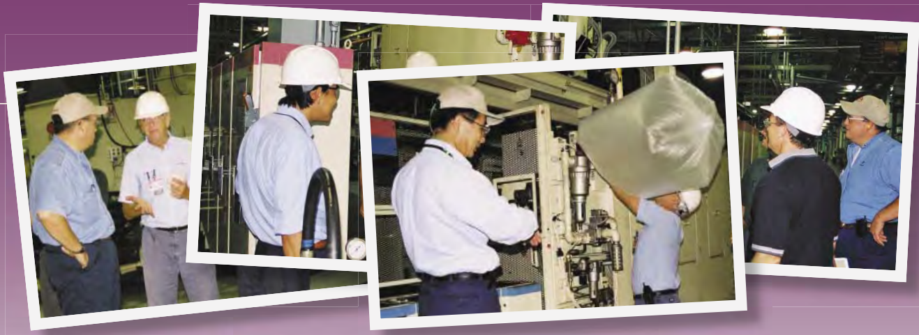
Hunting for energy-saving “treasures” began in 1999, and has resulted in over $9.2 million in savings. These hunts for energy reduction opportunities are conducted at two assembly plants and two unit plants each year. Above, team members measure compressed air leaks with a bag and timer during a treasure hunt at the manufacturing plant in Buffalo, West Virginia.
